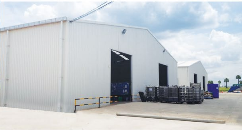
Warehouse CPF - Korat
